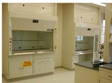
Figure 1: Flammable liquid storage cupboard below a fume hood
